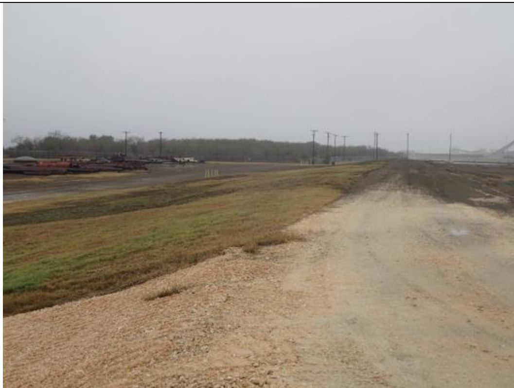
Photograph: 18 North Bottom Ash Pond – Outside of eastern berm. Photo taken 12/19/17.
