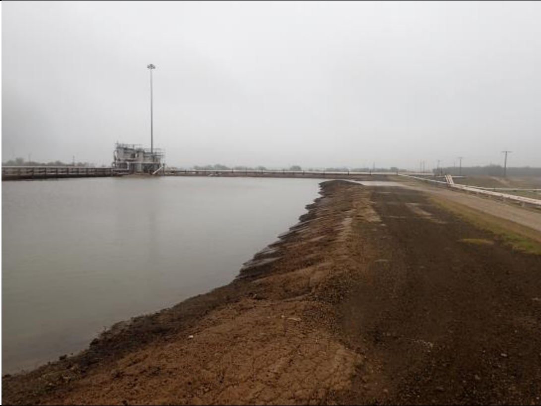
Photograph: 25 South SRH Pond – standing on southwestern corner – facing east. Photo taken 12/19/17.
