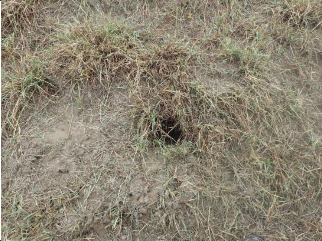
Photograph: 7 Fly Ash Landfill – standing on northern berm. Animal burrow in exterior slope. Photo taken 12/19/17.
