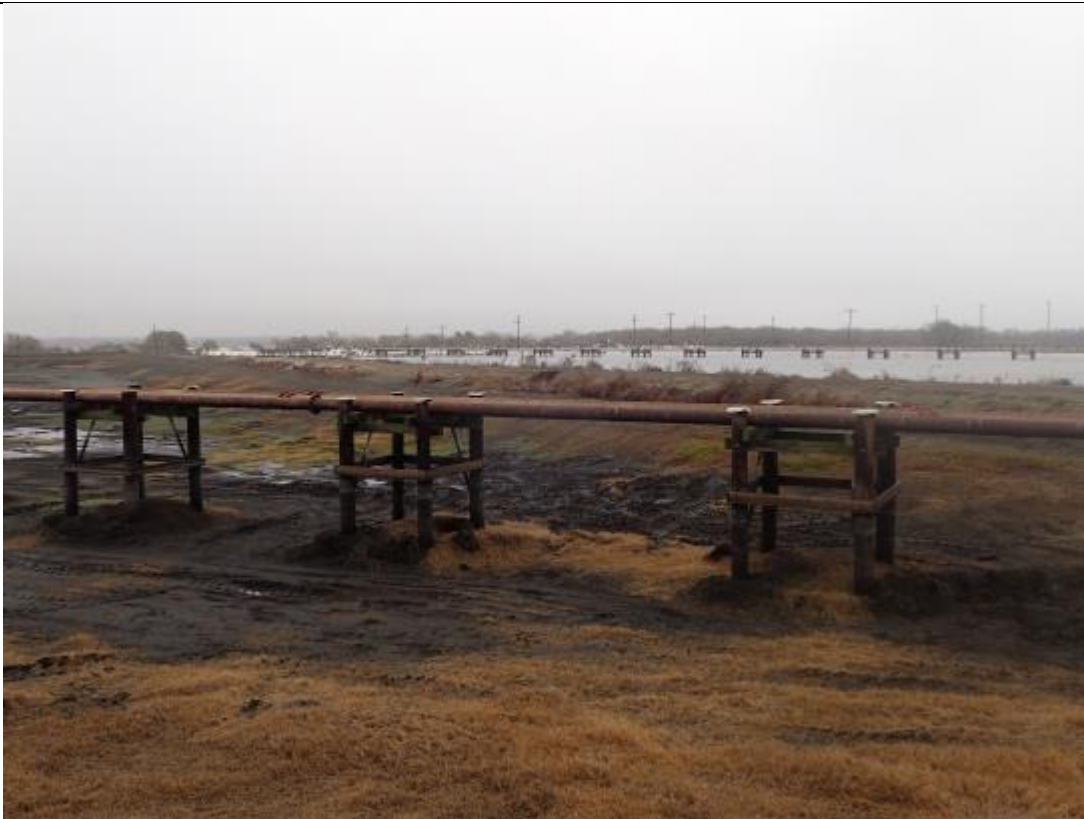
Photograph: 17 North Bottom Ash Pond – standing on northwestern berm – facing southeast. Photo taken 12/19/17.
