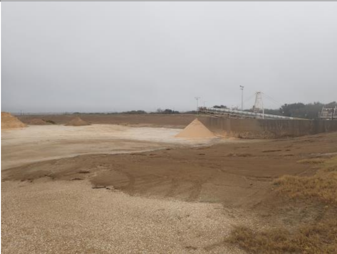
Photograph: 3 Fly Ash Landfill – standing on western berm – facing southeast. Radial stacker located in southwest corner of landfill. Photo taken 12/19/17.
