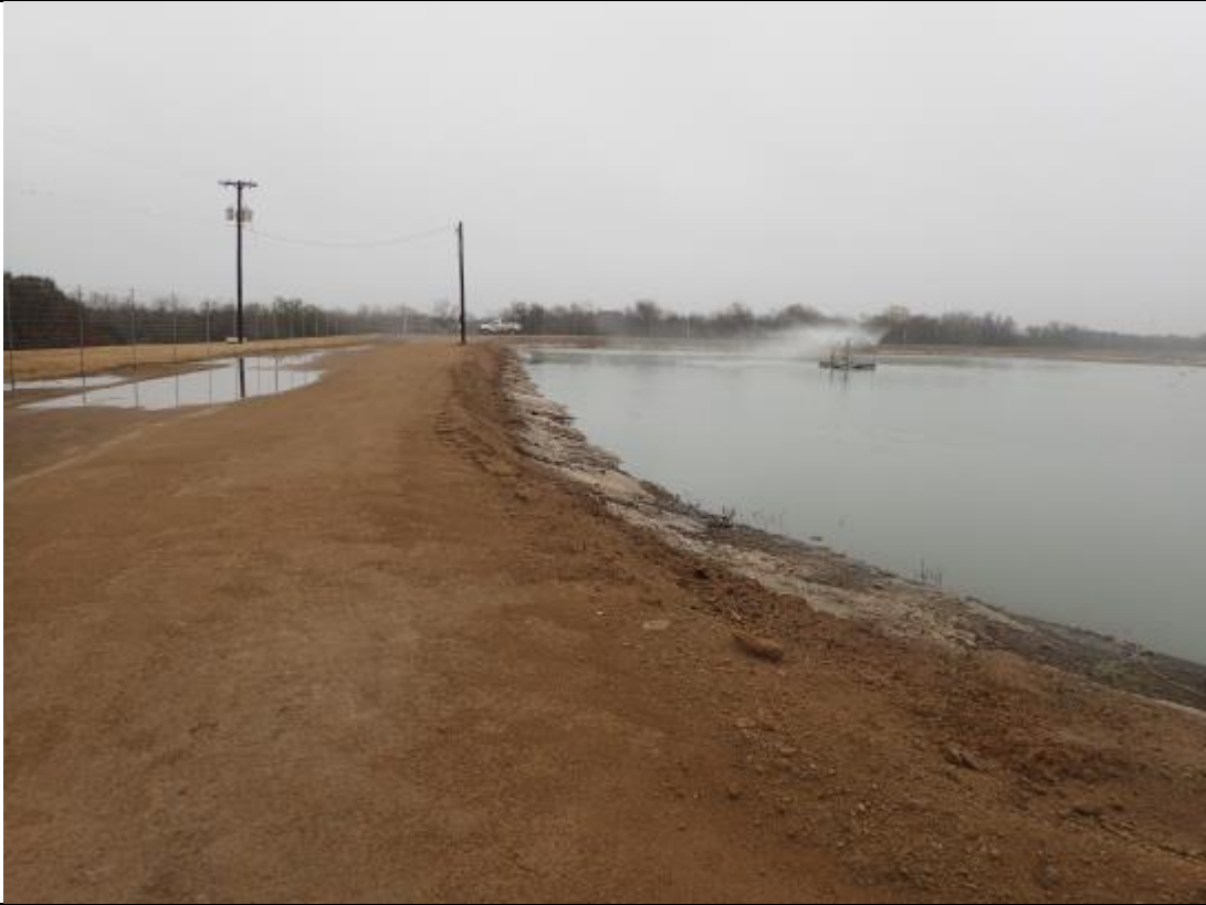
Photograph: 11 Evaporation Pond – standing on northwest corner – facing east. Photo taken 12/19/17.
