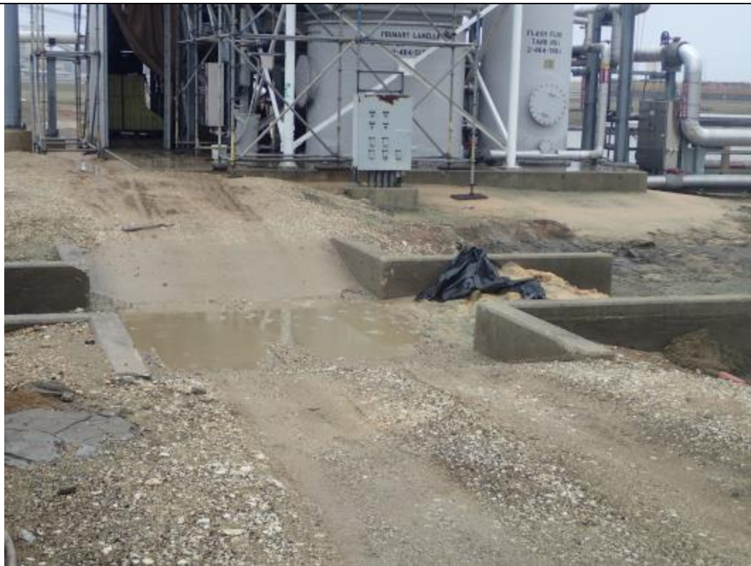
Photograph: 24 North SRH Pond – Overflow structure to South Bottom Ash Pond. Photo taken 12/19/17.
