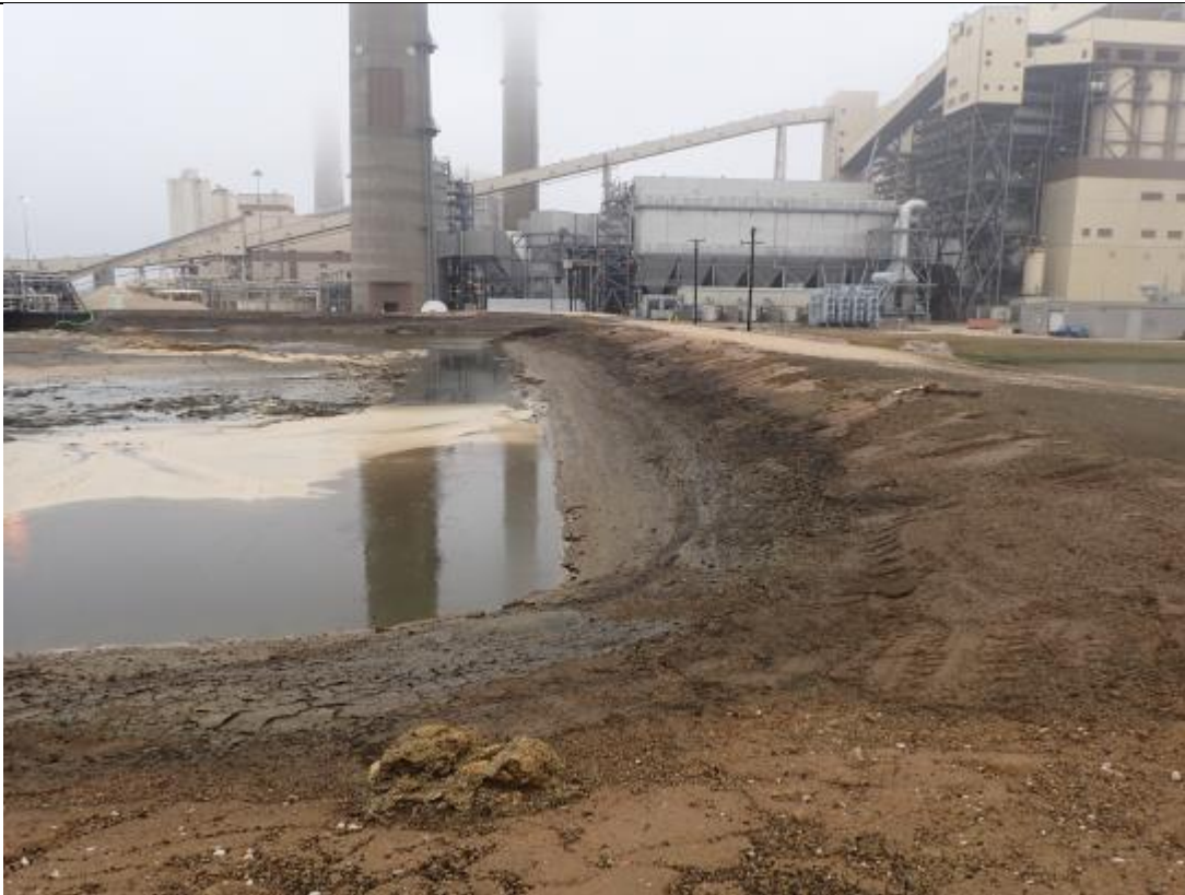
Photograph: 21 North SRH Pond – standing on northeast corner – facing west. Photo taken 12/19/17.
