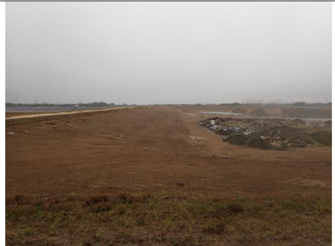
Photograph: 4 Fly Ash Landfill – standing on eastern berm - facing south. Photo taken 12/19/17.
