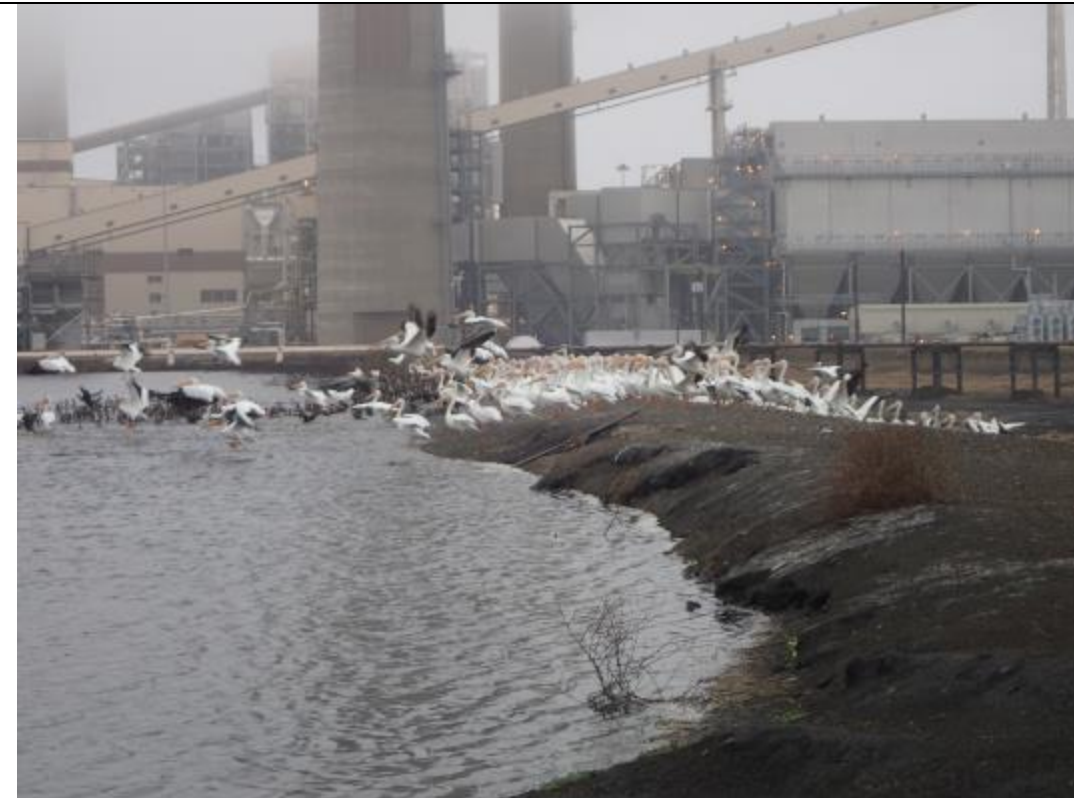
Photograph: 30 South Bottom Ash Pond – standing on northwest corner – facing west. Photo taken 12/19/17.
