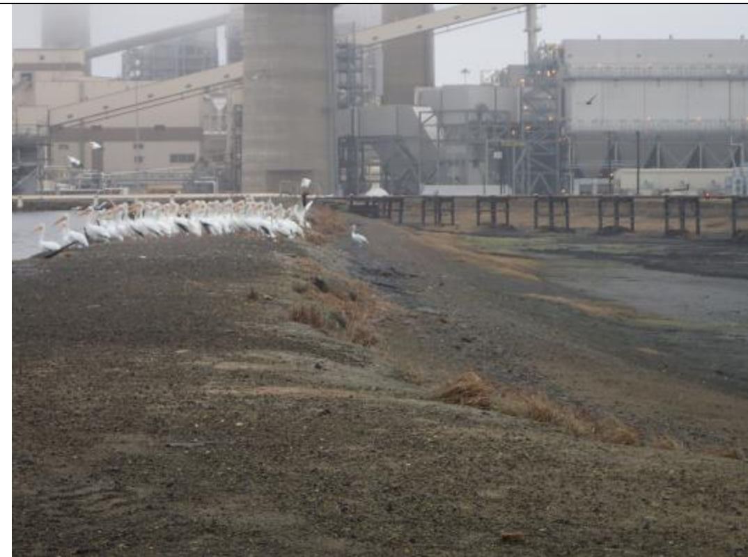
Photograph: 20 North Bottom Ash Pond – standing on southern berm – facing west. Photo taken 12/19/17.
