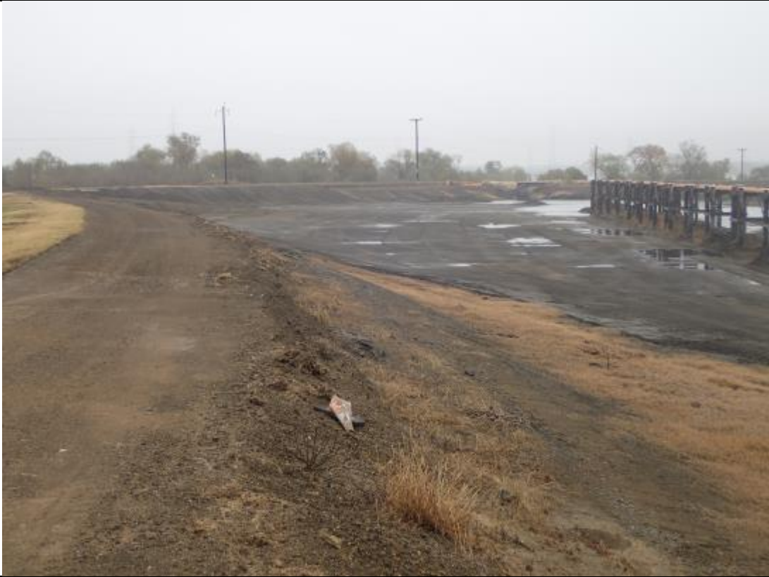
Photograph: 15 North Bottom Ash Pond – standing on southwestern corner – facing northeast. Pond was drained to remove residuals. Photo taken 12/19/17.
