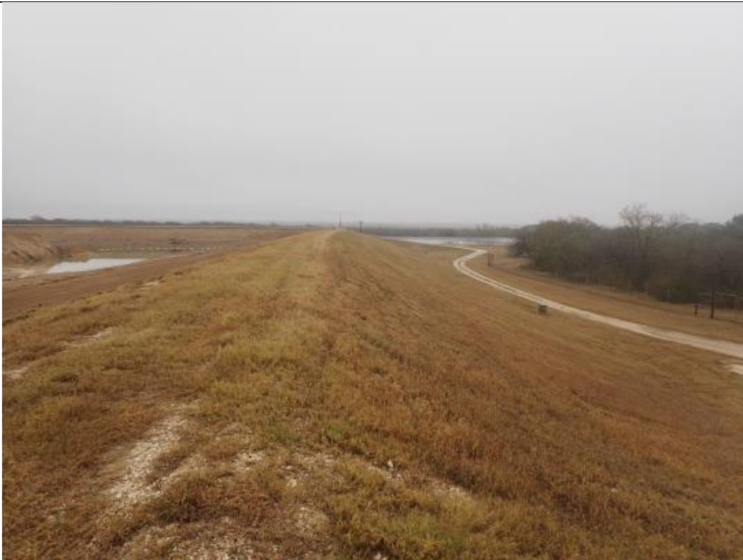
Photograph: 9 Fly Ash Landfill – standing on southern berm – facing east. Photo taken 12/19/17.
