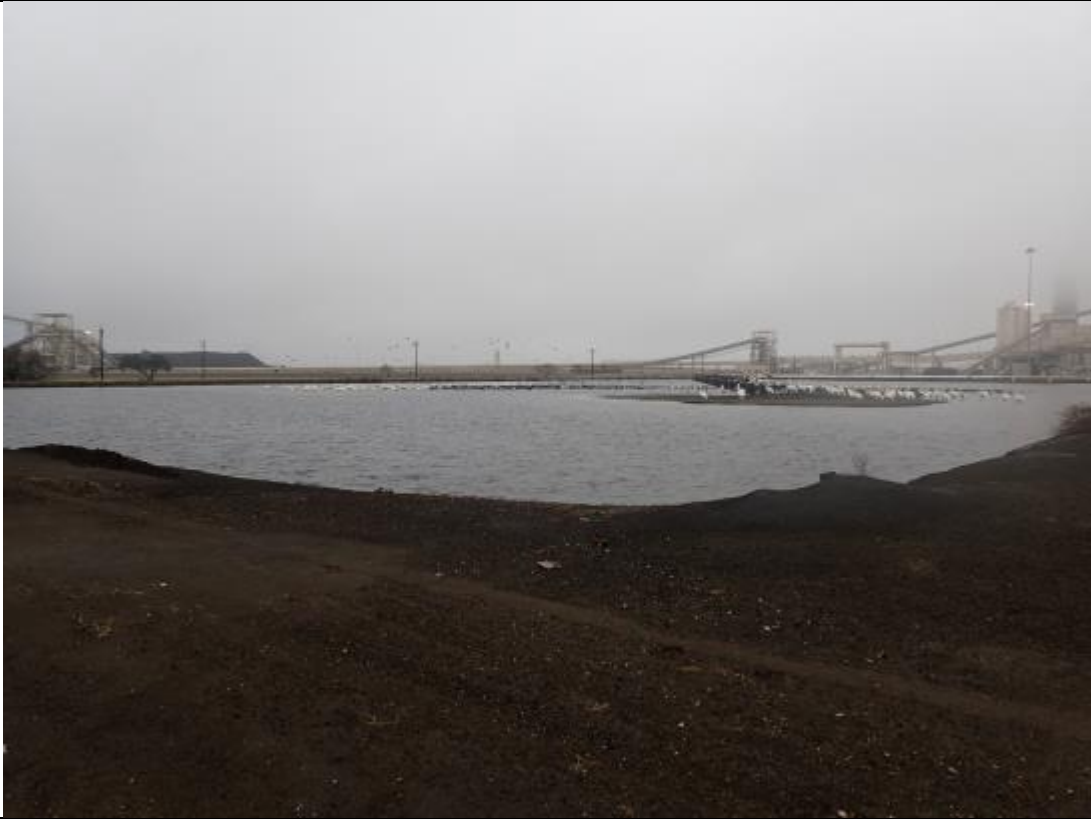
Photograph: 29 South Bottom Ash Pond – standing on northeast corner – facing southwest. Erosional features on eastern berm. Photo taken 12/19/17.
