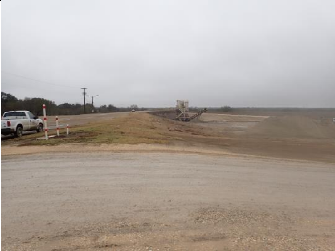
Photograph: 1 Fly Ash Landfill – standing on western berm – facing north. Mobile ash conditioning machine located in northwest corner of landfill. Photo taken 12/19/17.
