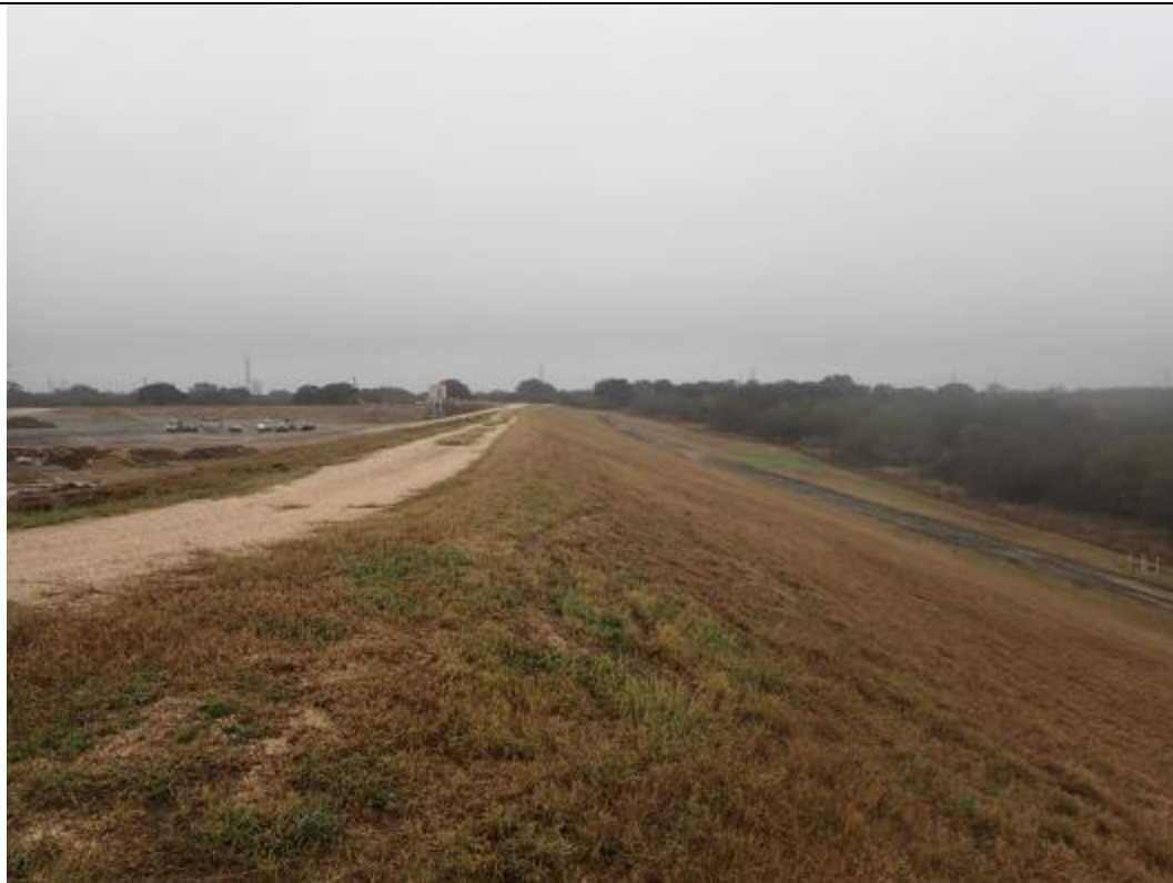
Photograph: 6 Fly Ash Landfill – standing on northern berm – facing west. Photo taken 12/19/17.
