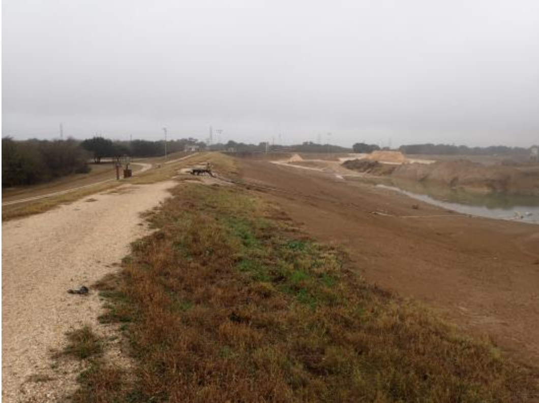
Photograph: 8 Fly Ash Landfill – standing on southern berm – facing west. Photo taken 12/19/17.
