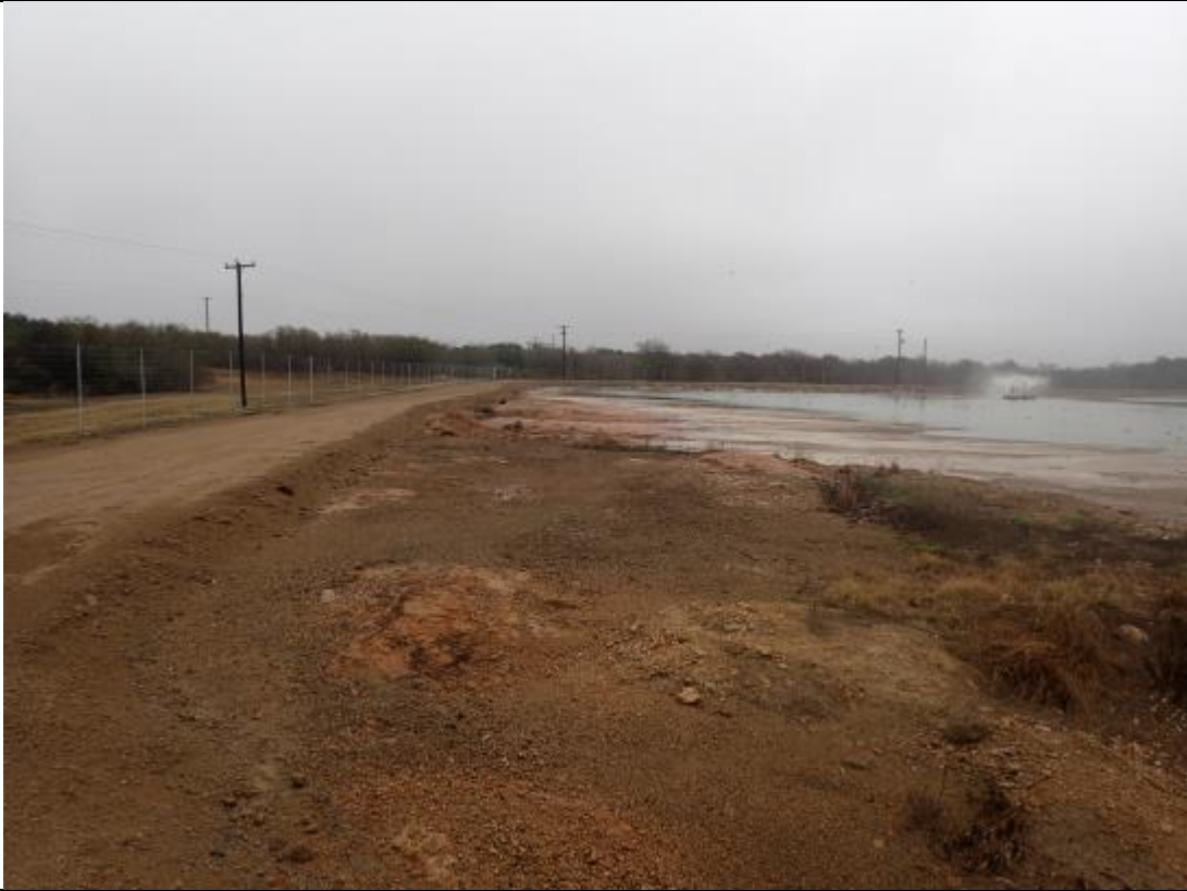
Photograph: 13 Evaporation Pond – standing on southwest corner – facing north. Photo taken 12/19/17.
