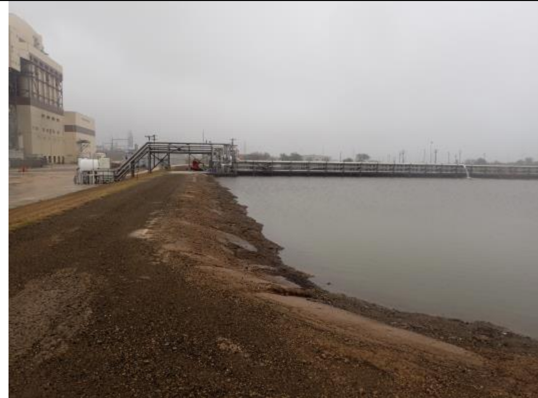
Photograph: 26 South SRH Pond – standing on western berm – facing north. Photo taken 12/19/17.
