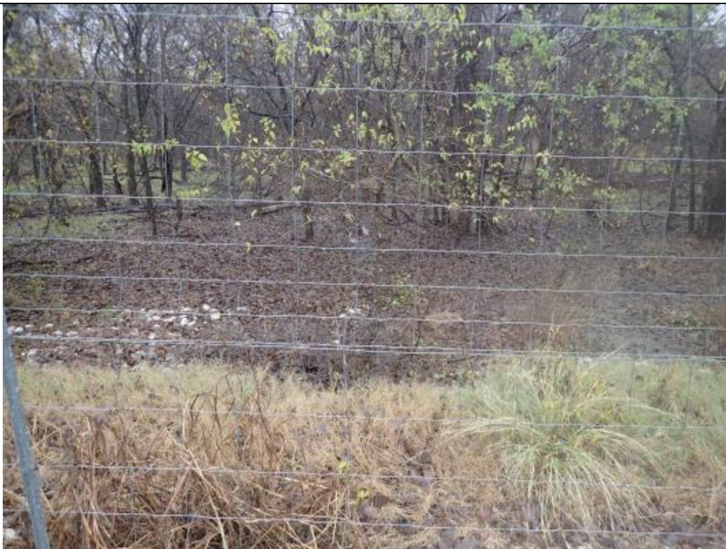
Photograph: 10 Fly Ash Landfill – outside eastern perimeter at northeast corner drainage discharge. Photo taken 12/19/17.
