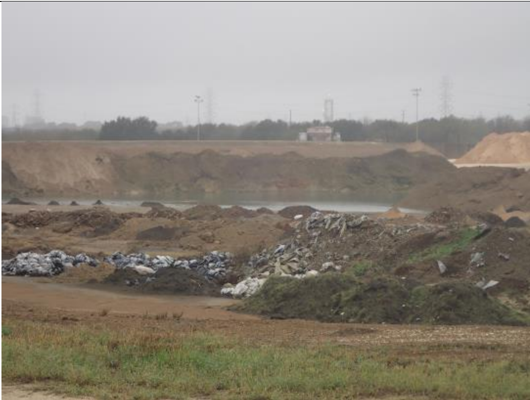
Photograph: 5 Fly Ash Landfill – standing on eastern berm – facing southwest. Water accumulation from recent rain events. Photo taken 12/19/17.
