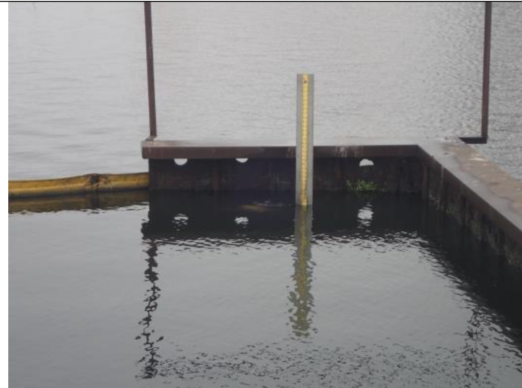
Photograph: 28 South Bottom Ash Pond – Outfall structure. Photo taken 12/19/17.
