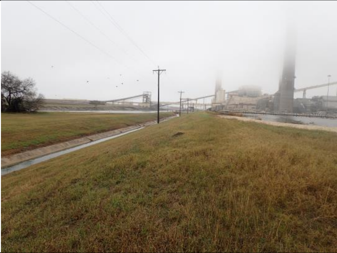
Photograph: 27 South Bottom Ash Pond – standing on southeastern corner – facing west. Photo taken 12/19/17.
